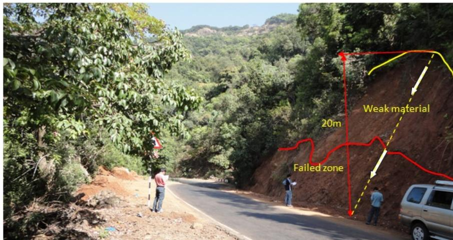
**Figure 2.** The cut slope along the road cut on SH-72, near Mahabaleshwar, India.
